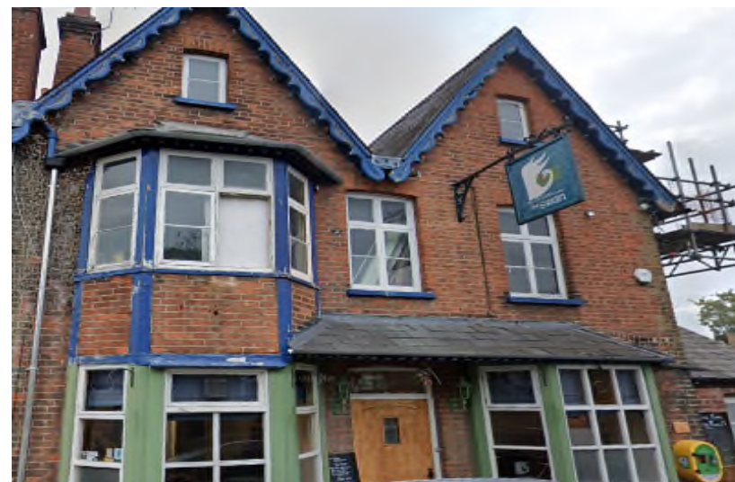
Fig. 53 Frontage of The Swan public house
