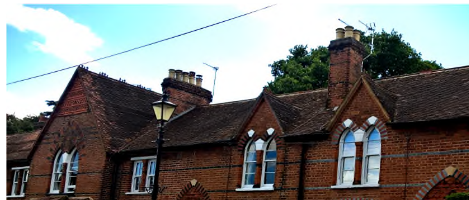
Fig .68 15-35 Mill Lane, gables and chimneys with terracotta chimney pots
