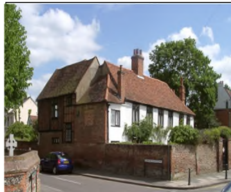
Fig. 91 The Limes viewed from Mill Lane
