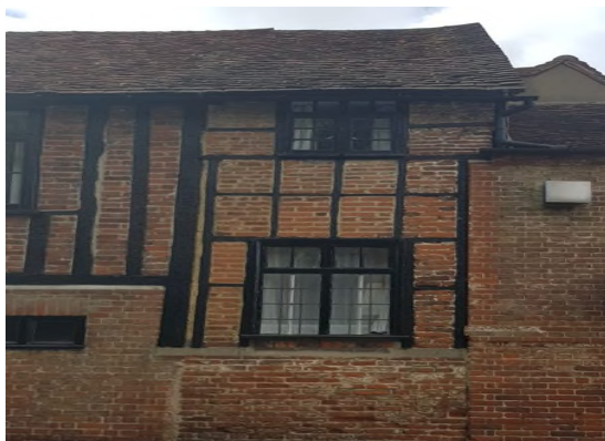
Fig. 50 The Limes, exposed timber framing to northern elevation
