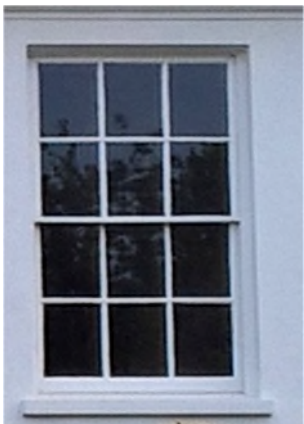
Fig. 70 Edgeworth House, Georgian sash window with early glass and fine glazing bars
