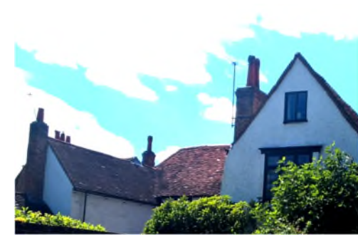
Fig. 67 The roof of the Limes has weathered hand made clay tiles
