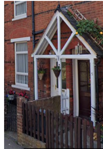
Fig. 77 Shared pitched roof open porch over 3/5 Mill Lane
