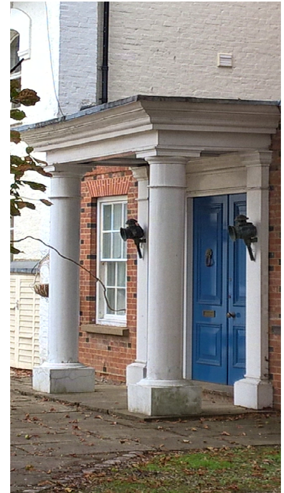
Fig. 79 Old Mill House, Georgian timber door with deep mouldings and raised and fielded panels, under a porch supported on Doric columns
