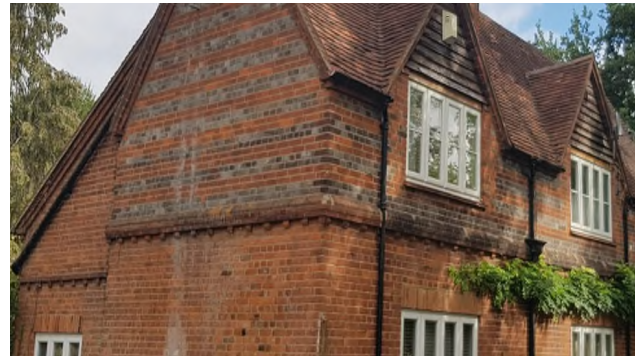
Fig. 58 projecting and moulded brickwork banding and use of polychromatic brickwork on the upper floor of Riverside
