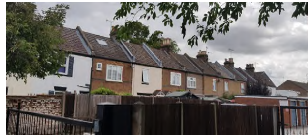
Fig 55 the south elevation of Swan Terrace with numerous alterations
