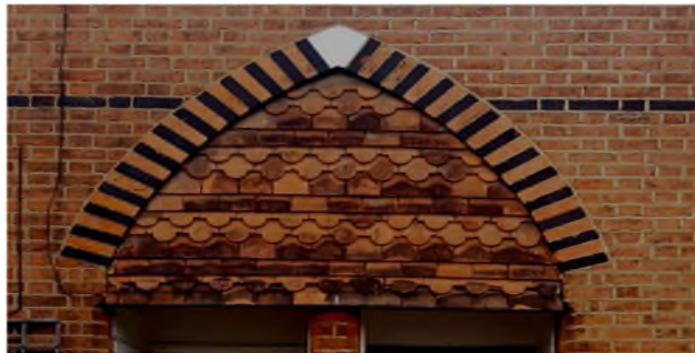
Fig. 59 bull nose and fishtail pattern tile hanging, and decorative brick and stonework detailing on one of the Victorian terraces
