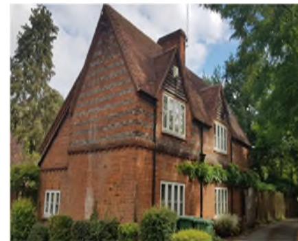
Fig. 101 Riverside, Mill Lane
