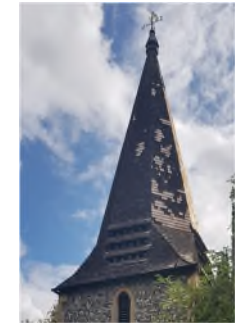
Fig .65 St Andrews Church, spire clad in timber shingles
