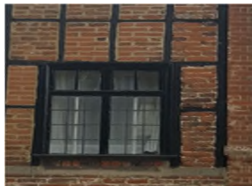
Fig. 71 The Limes, metal and timber casements with leaded lights
